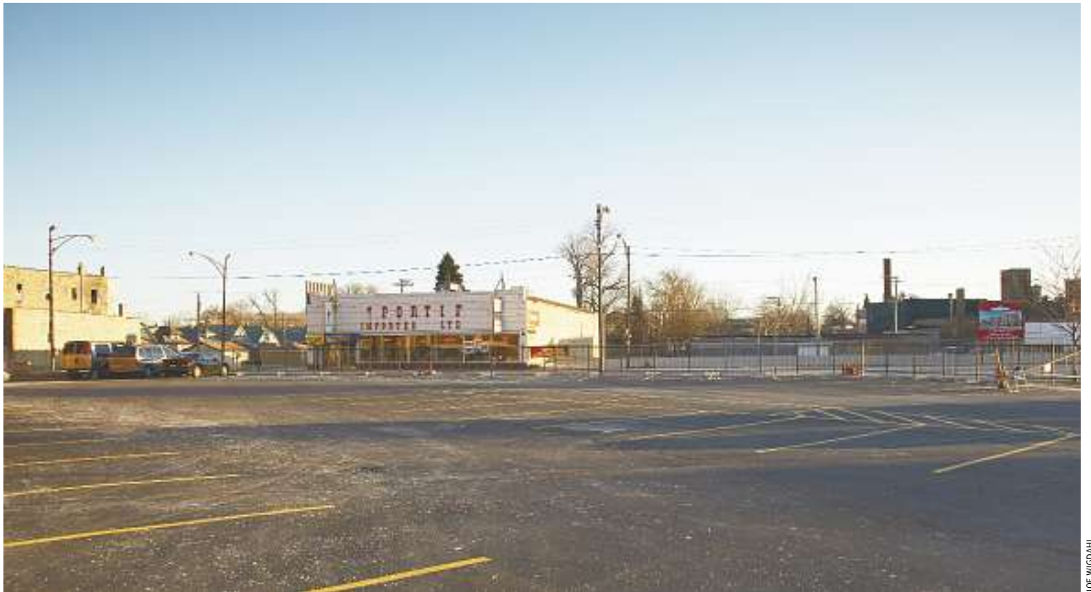
Sportif bike store, on the 5200 block of West Lawrence
